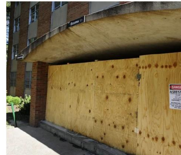
Stephen Ricker / The Southern Boomer Hall is sits boarded up and asbestos warnings have been posted as the resi awaits demolition this summer.
