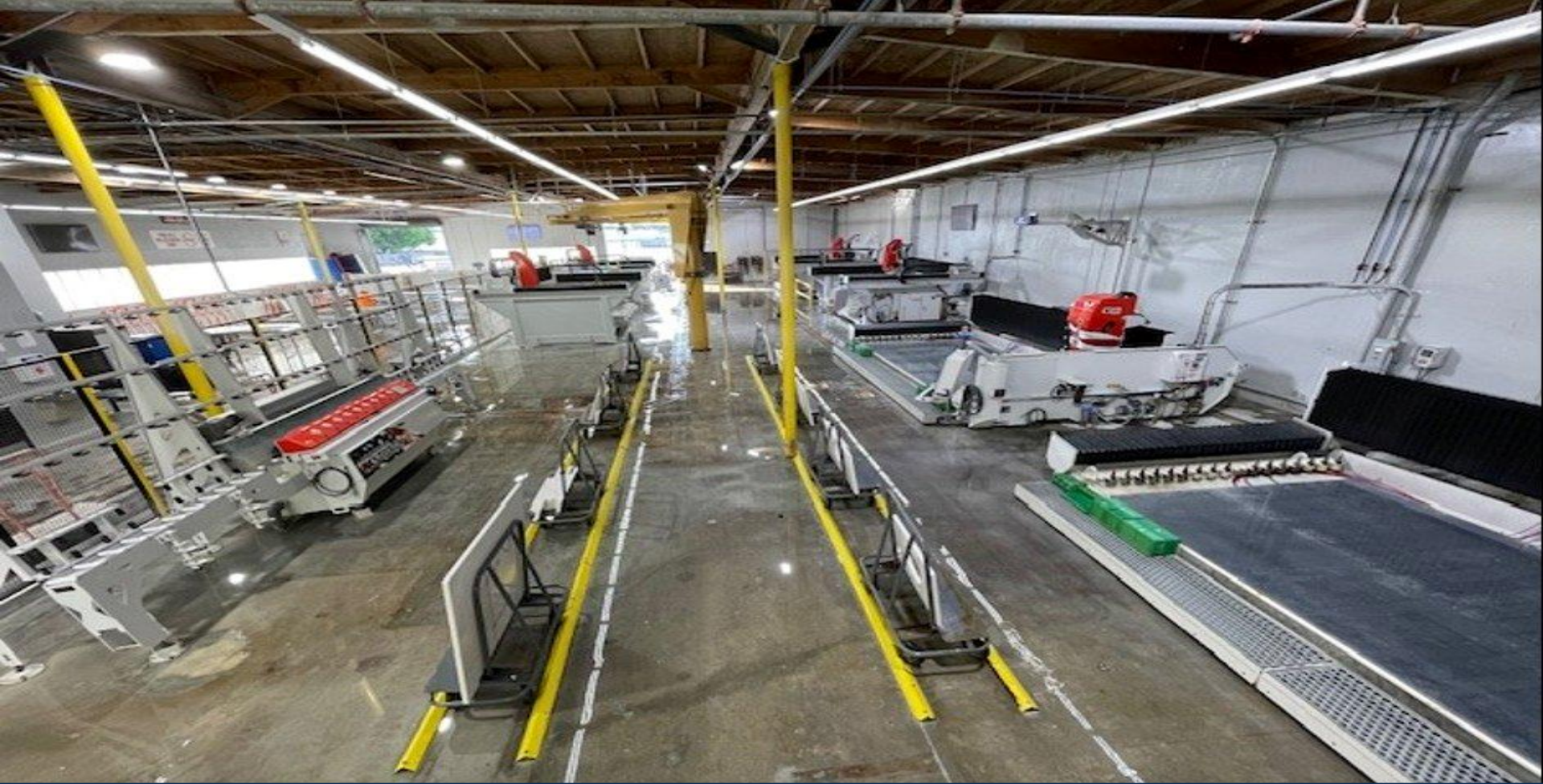
Aegean Stoneworks — Production floor: automated CNC bridge saws, routers, inline edger, and sawjet wet system.
